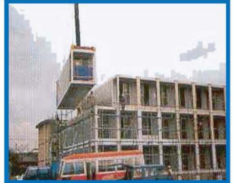
INSTALLATION AT SITE
