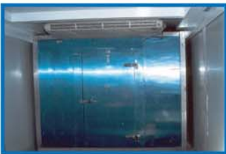
COLD STORAGE ROOM
